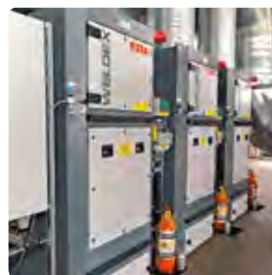
Several WELDEX F-100 filter modules for a central extraction system. Extinguishing system as an optional accessory
